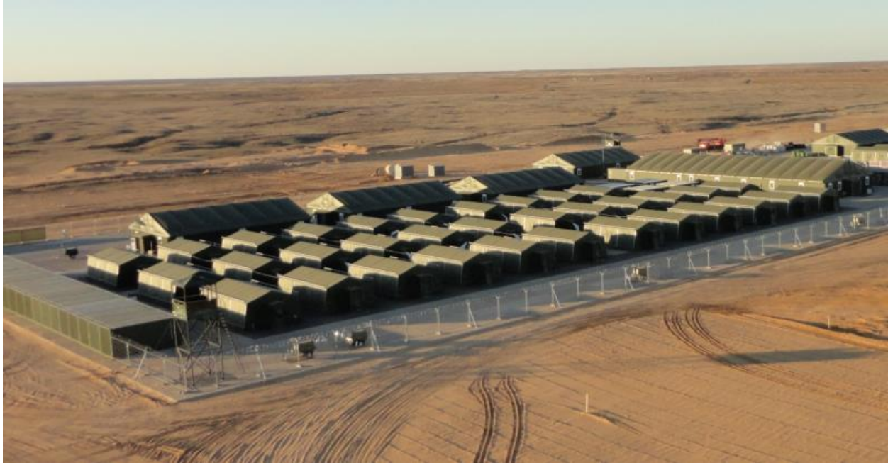
Living quarters, chow hall, training and counseling space, bathrooms, and perimeter security.
